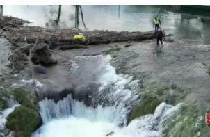
The small branches could be easily detached with a hook and washed away by the river current. At one point the branches were removed with a fire.
