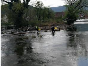
In addition to small branches, there were also large tree trunks, which meant that the river could not flow unhindered and had to find its way around the hill of branches. A rope was attached to the large tree trunks so that a tractor could pull most of them out. When they reached the shore, the thick logs were cut up by hand with a chainsaw and then pulled out.
